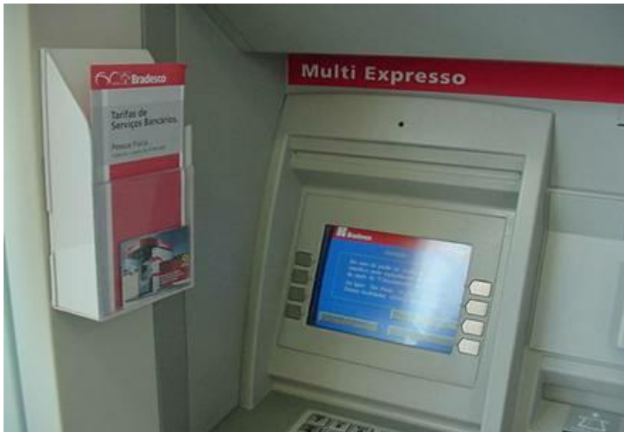
The camera shown installed and ready to capture PIN's by looking down on the keypad as you enter your PIN
